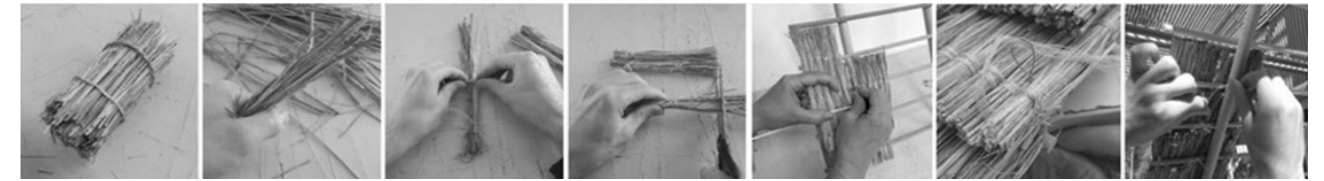
Operating chain 2: From bale to row (wall, roof). A. Coscolluela, B. Houllis, ©LMdP 2022.
