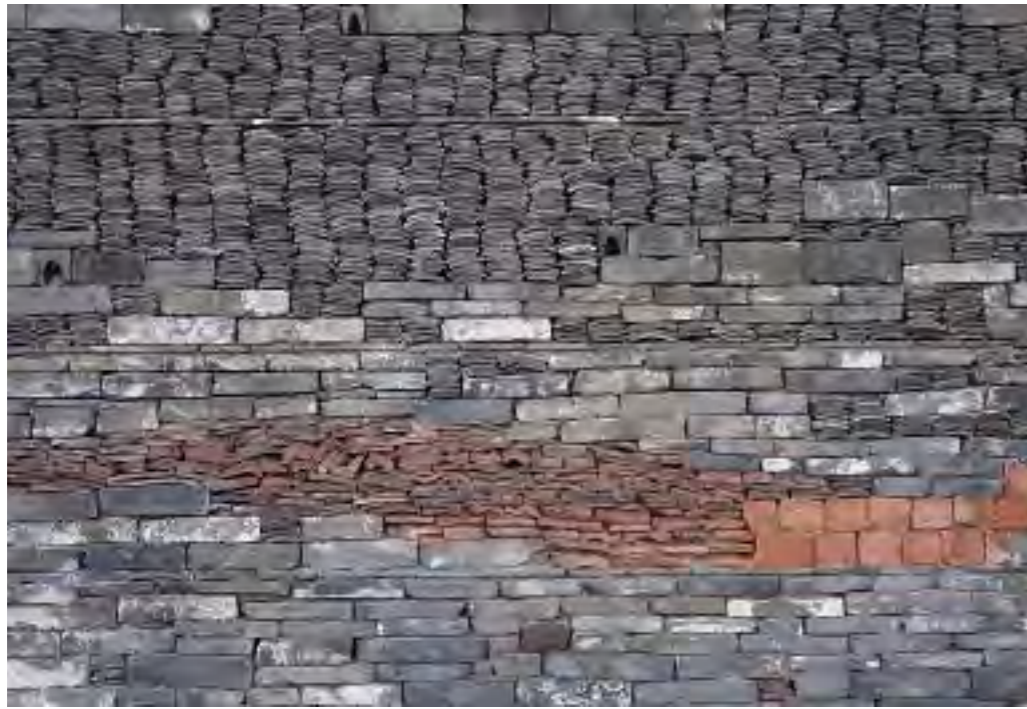
Figure 2. Wapan wall (source: Siyuwj, the building designed by Wang Shu, CC BY-SA 3.0 < https://creativecommons.org/licenses/by-sa/3.0/ >, via Wikimedia Commons)
