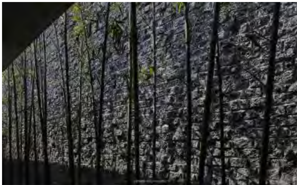
Figure 6. Recycled brick in Shuijingfang Museum. (Source: Jiakun architect < http://www.jiakun.com/project/detail?id=11 >)
